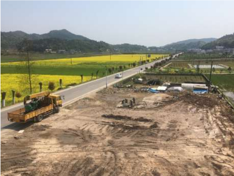
Figure 1. High-tech farm under construction in rural Hunan. Photograph by Ettore Santi, 2018.
